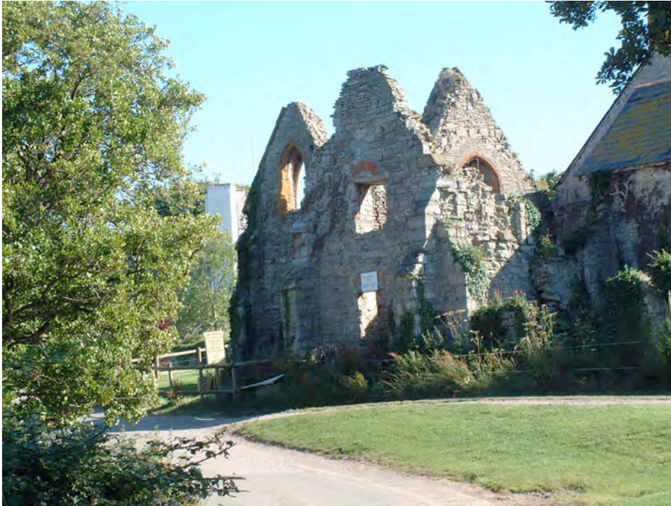
The Chantry before restoration work started
