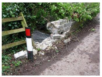
The bridge at the junction of Hilltop Lane and Sea Lane has suffered major impact damage to the parapet – farm tractors and trailers are believed to be the cause. It was restored in late 2021 and then had identical damage only a few weeks later. The masonry has fallen into the stream, now posing a safety risk to pedestrians (particularly to the disabled and partially sighted) as the 2m drop into the concrete base of the stream is now unguarded for a width of about 1m.
